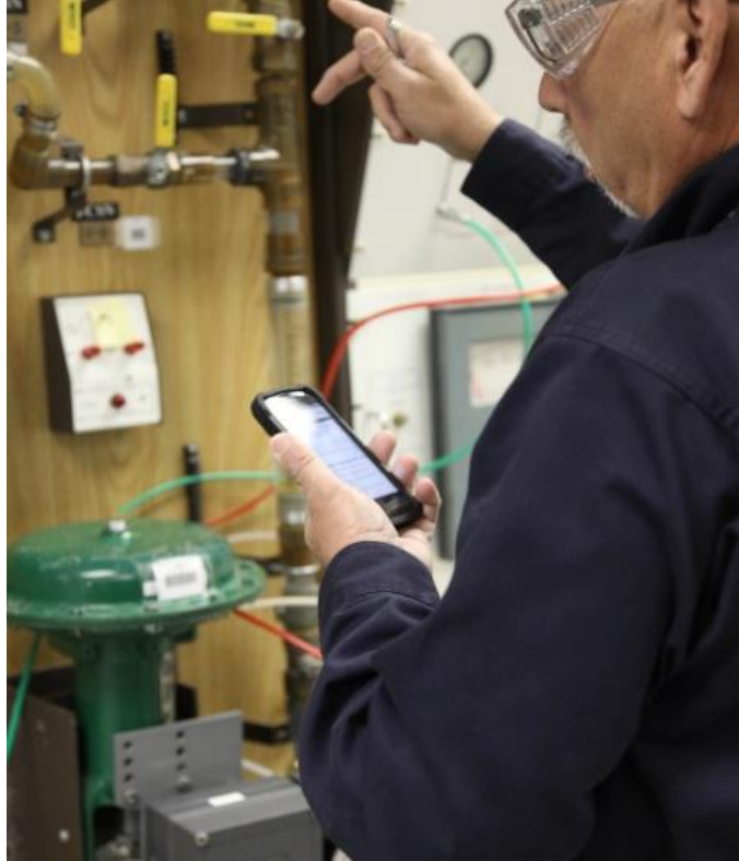
Figure 9. A field worker at Palo Verde Nuclear Generating Station uses the CBP to execute a task.
