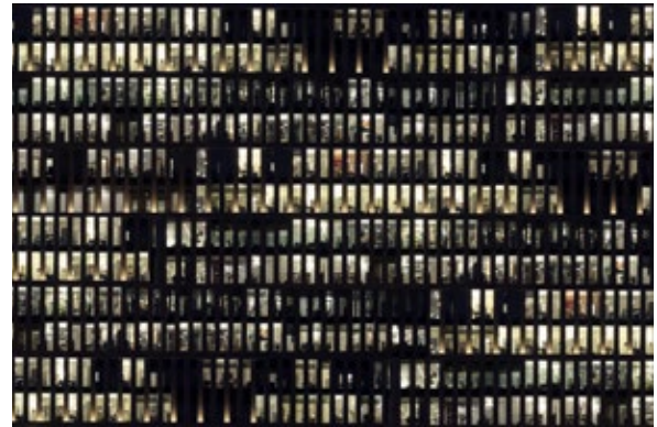
FIGURE 41 Reflective glazings prevent view of interiors from the outside during the day, as the reflected radiation is significantly higher than that transmitted from the interior light levels. However, they allow a clear view of interiors during the night when the electric lights are on. The opposite is true for an outdoor view from the inside of the space.
