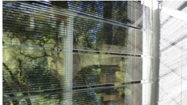
FIGURE 48 Photograph of light redirecting microstructure installed on a window, showing the direct and redirected patterns on the transmitted radiation on the side wall of the space.
