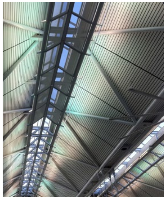
FIGURE 26 Linear skylights with sloped glazing.
