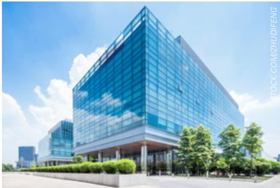
FIGURE 41 Reflective glazings prevent view of interiors from the outside during the day, as the reflected radiation is significantly higher than that transmitted from the interior light levels. However, they allow a clear view of interiors during the night when the electric lights are on. The opposite is true for an outdoor view from the inside of the space.
