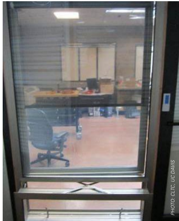
FIGURE 57 Photograph of shading systems between glazing panes.
