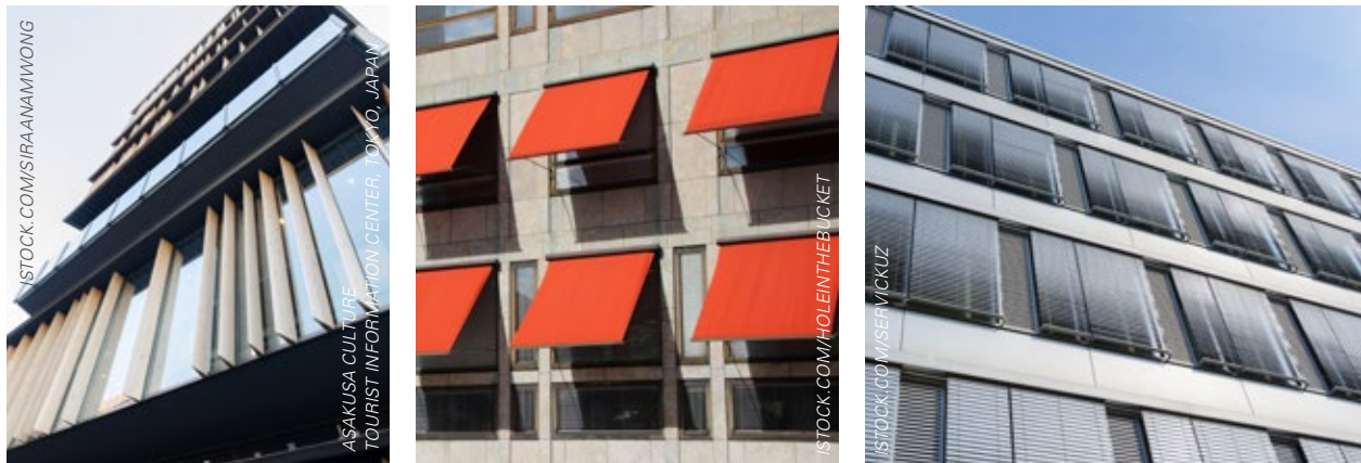
FIGURE 51 Photographs of building facades with exterior shading systems.
