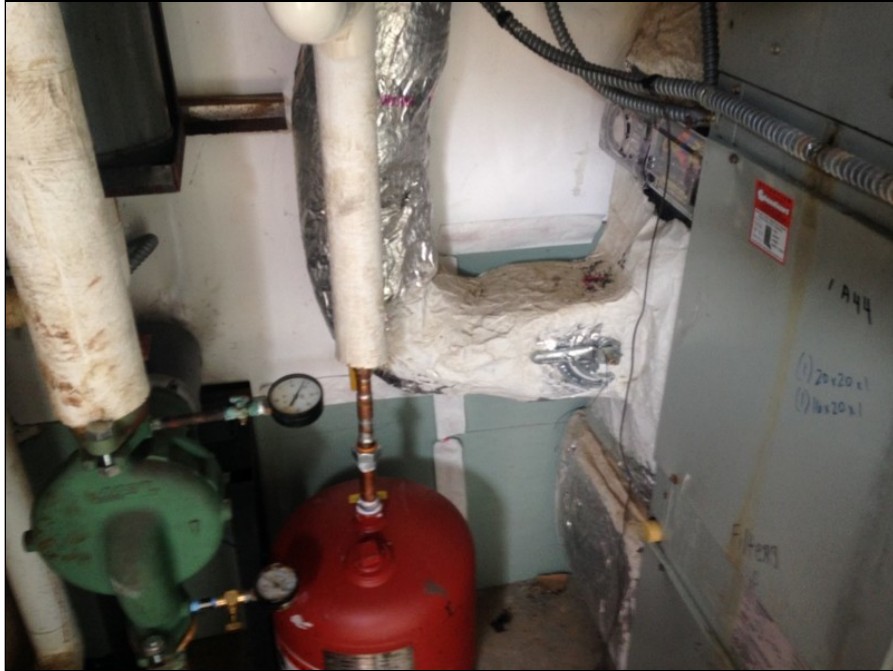
15 - View of HVAC Mastic
