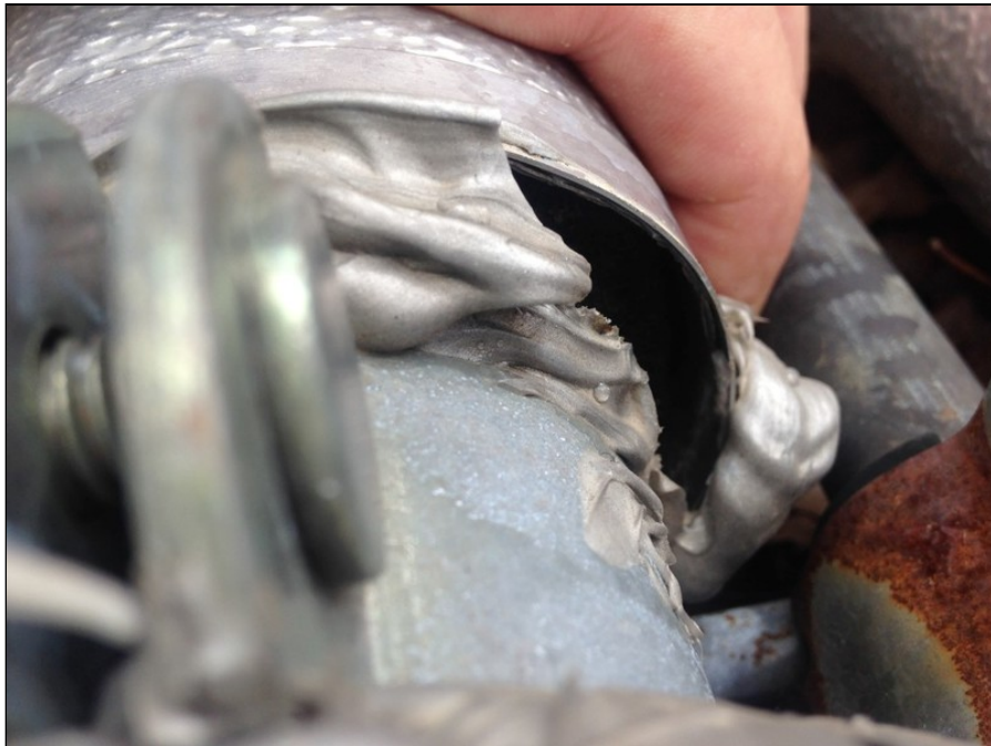
14 - View of HVAC Mastic
