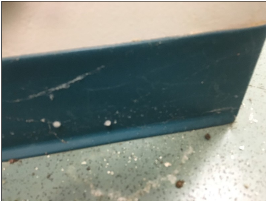
4 - View of the green cove base (Sample 02) located throughout the structure
