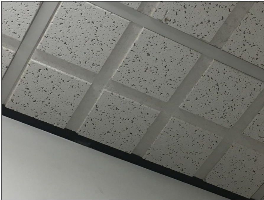
6 - View of the ceiling tile (Sample 06) located throughout the structure
