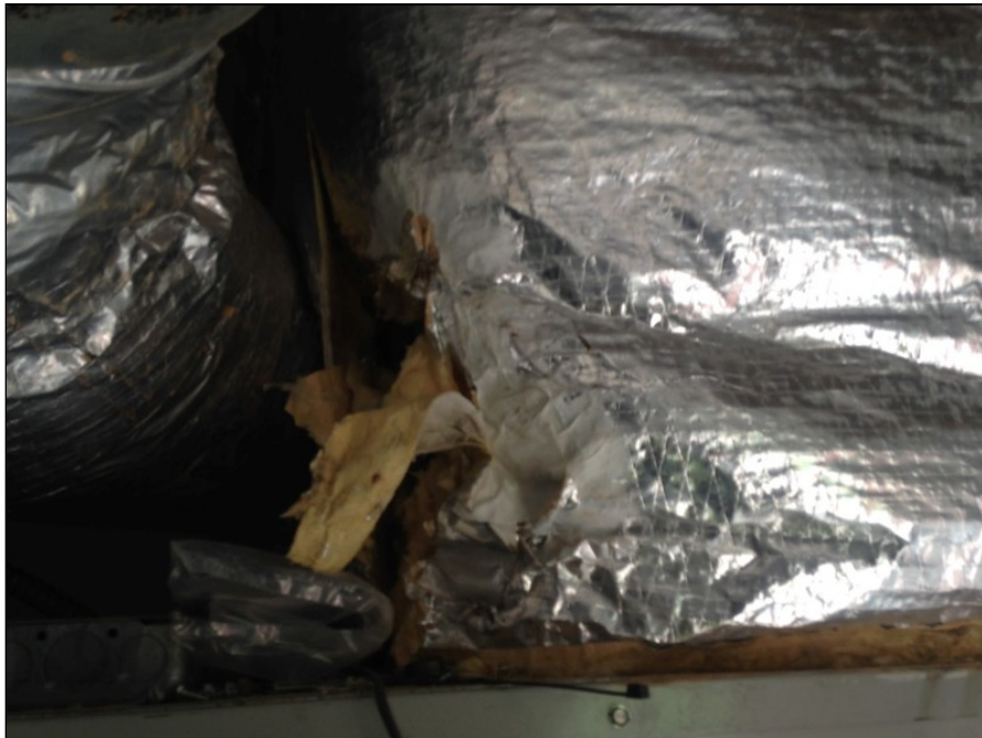
10 - View of HVAC Mastic (Sample 08)
