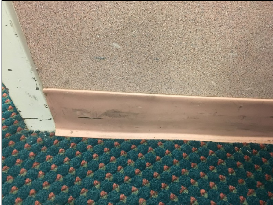
7 - View of the pink cove base (Sample 07) located throughout the office area
