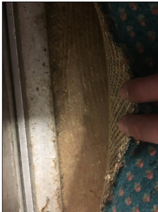
8 - View of the carpet and mastic (Sample 09) located throughout the structure
