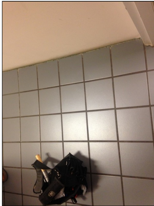
12 - View of beige ceramic tile in the kitchen area - Lead Based Coating
