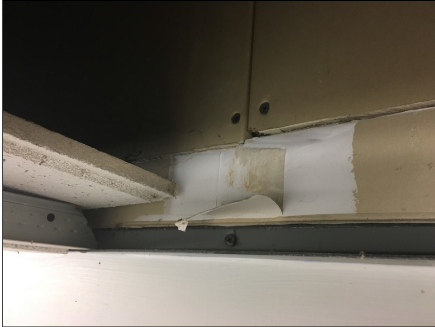
3 - View of Drywall/Joint Compound (Sample 01) above the drop ceiling
