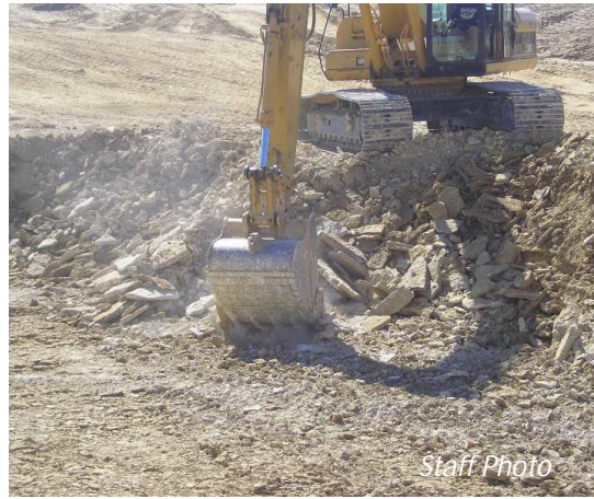
Figure 5: Photo of bedrock removal
