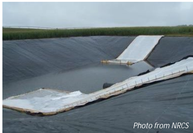
Figure 7: Concrete ramp on top of HDPE (note geo-textile between concrete and HDPE)
