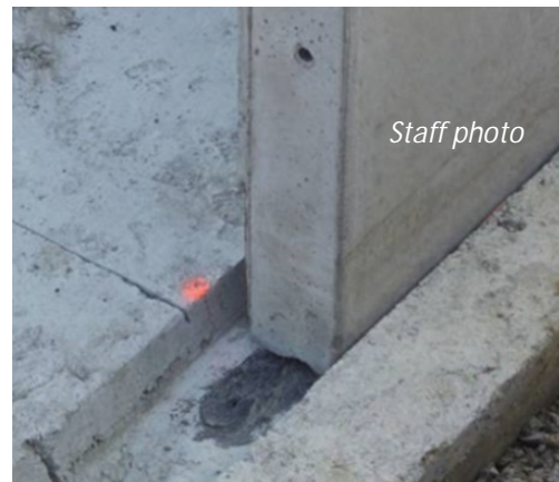
Figure 10: Floor keyway for pre-cast concrete wall panels
