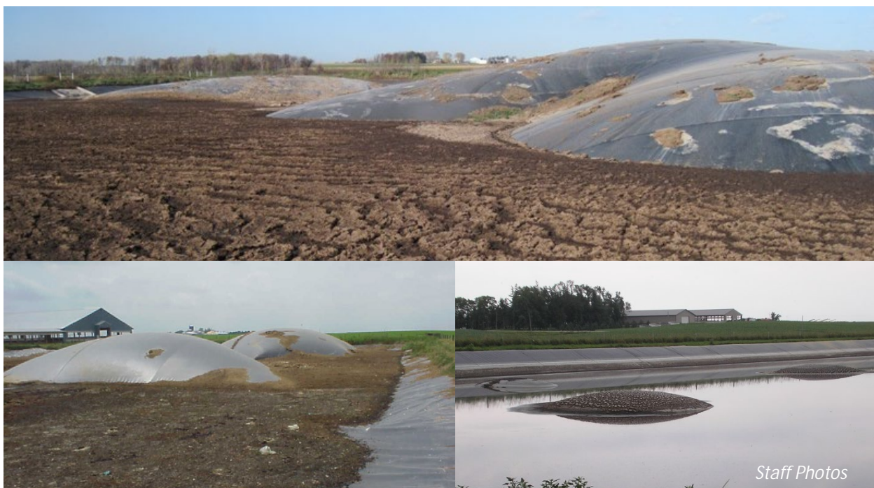
Figure 8: Photos of “whales” (trapped pockets of bio-gas) within plastic lined LMSAs
