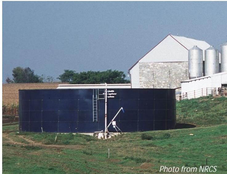
Figure 9: Photo of a typical steel above ground LMSA
