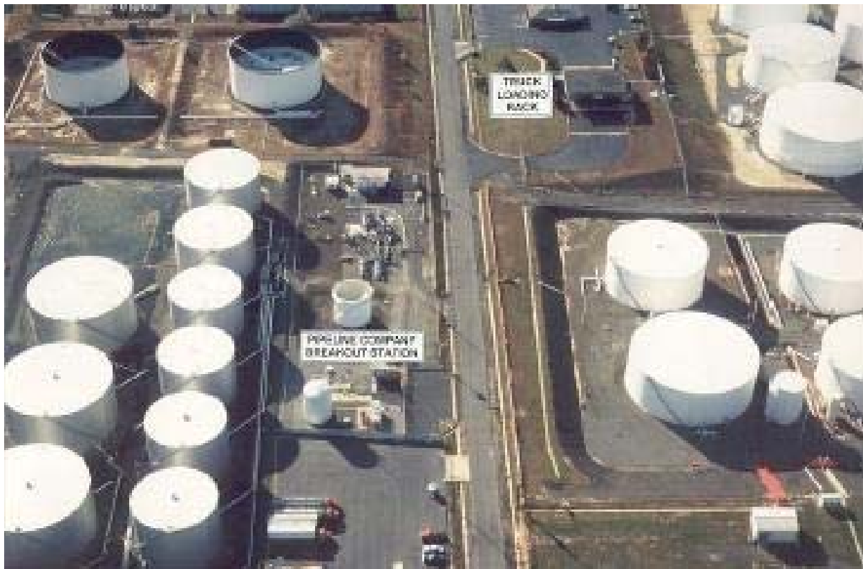
FIGURE 3.3-27 Typical Pipeline Breakout Station (Terminus) at a Petroleum Terminal (Source: V. Yarborough, Argonne staff)
