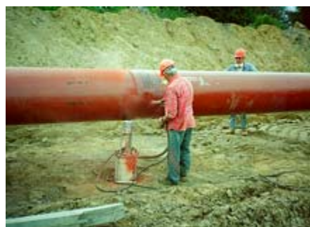
FIGURE 3.3-12 Applying Coating to Pipeline
