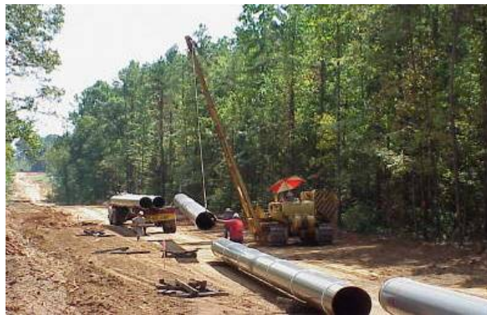
FIGURE 3.3-7 Stringing Pipe along the ROW (Source: Photo courtesy of U.S. Pipeline, Inc. Reproduced with permission.)
