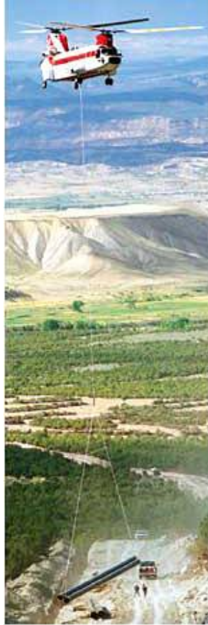
FIGURE 3.3-8 Delivering Pipe Segments to the Construction Site in Rugged Terrain May Require Special Equipment (Source: Photo courtesy of U.S. Pipeline, Inc. Reproduced with permission.)
