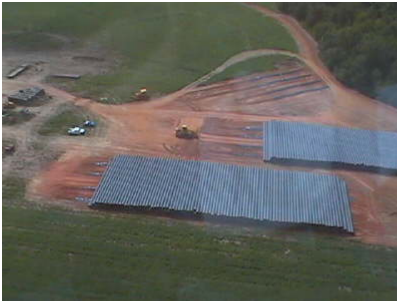
FIGURE 3.3-5 Pipe Segments in a Material Laydown Area (Source: Photo courtesy of U.S. Pipeline, Inc. Reproduced with permission.)
