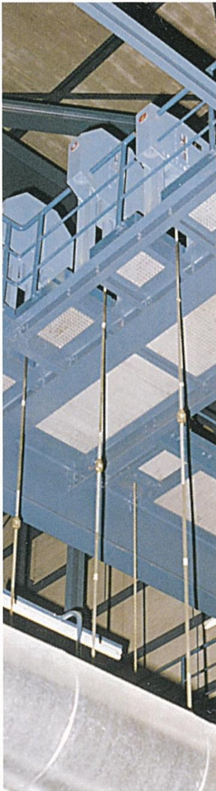
LISEGA constant hangers installed
