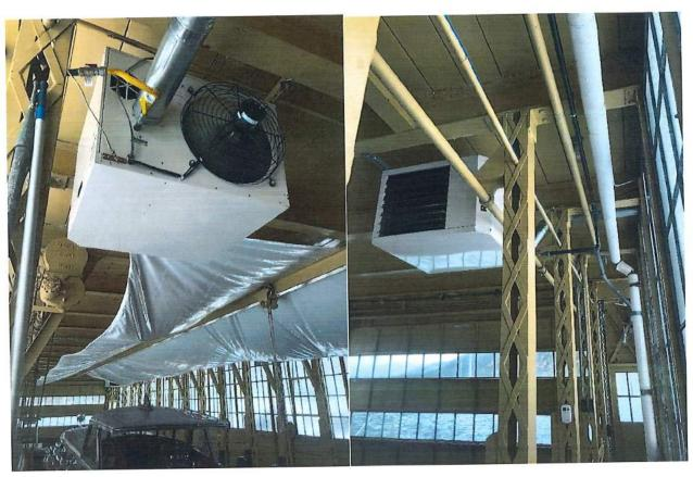
Plimpton Installed Dual State-of-the-Art Reznor Units with new electrical, gas supply, and venting, while Nevada 36 Companies Inc. supplied material and installed hangars, conduit, and control circuits.
