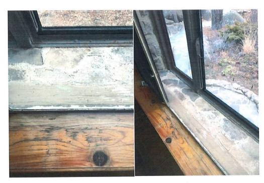
Close-up Detail of Air-Gap Area. Note grout will require replacement.
