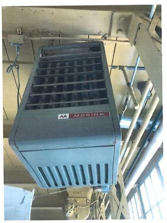
Non-vented, ungrounded, non-compliant 1970s era heater being replaced.
