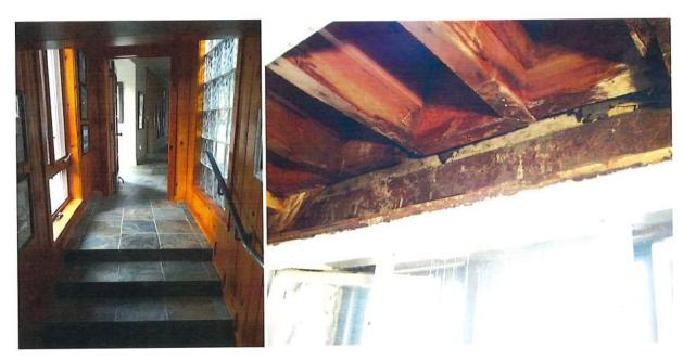
Connector Interior. Glass Block and Ceiling Leaking. Window unit on left has failed.
