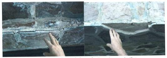
Failing masonry on underside of upper balcony due to water penetration.
