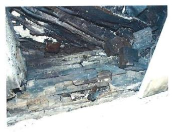
Opening-up the space beneath the leaking Old Lodge Door units reveals extent of damage.
