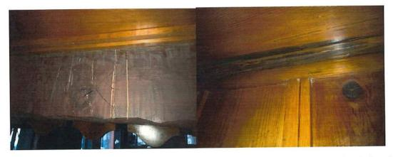
Water Passes Through Balcony Stone to Interior Spaces, below. Mold and Mildew is forming, not to mention what we will find in spaces behind the wall and ceiling boards.
