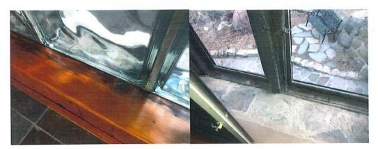
Water seepage under 1930s glass window block onto sills.
