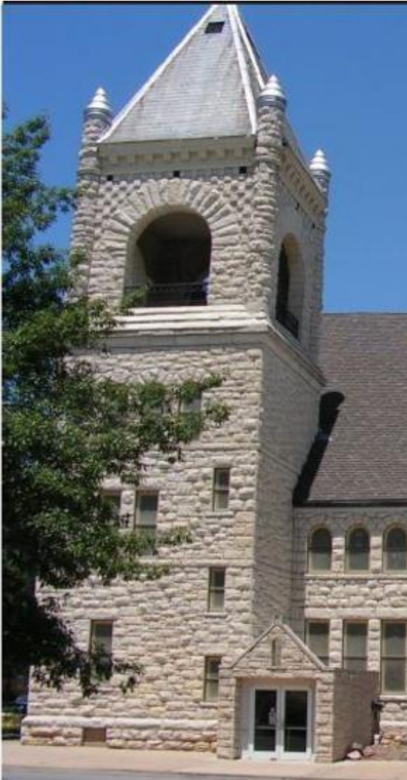
Figure 13: Entry and stairwell to old fellowship hall
