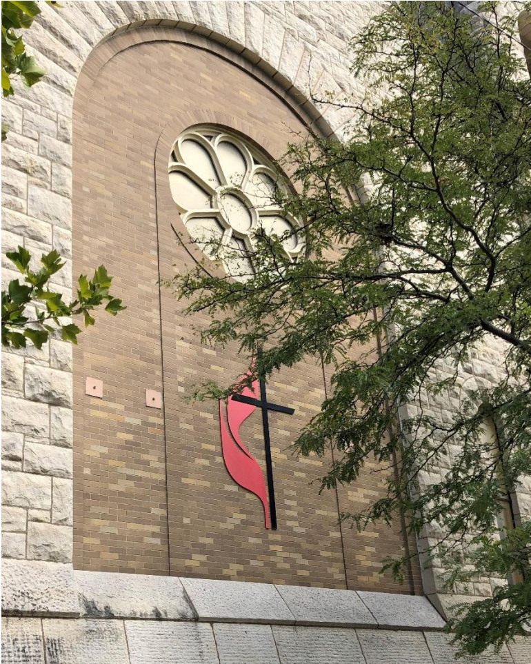
Figure 6: Former arch window
