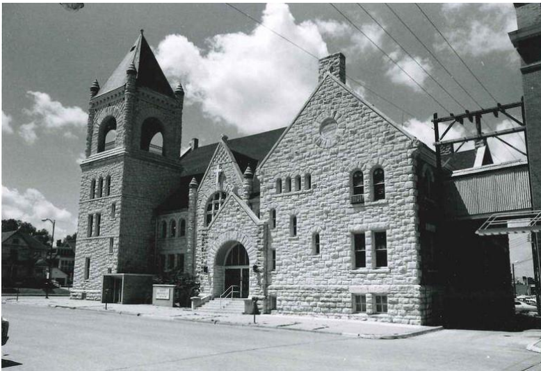
Figure 27: Bridge across alley, date unknown (between 1968 and early 1980s)
