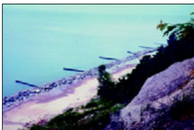
Groin and revetment system near St. Joseph, Michigan, on Lake Michigan
