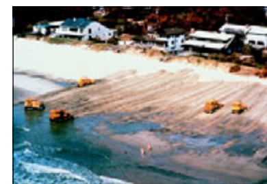
Beach nourishment along Lake Michigan
