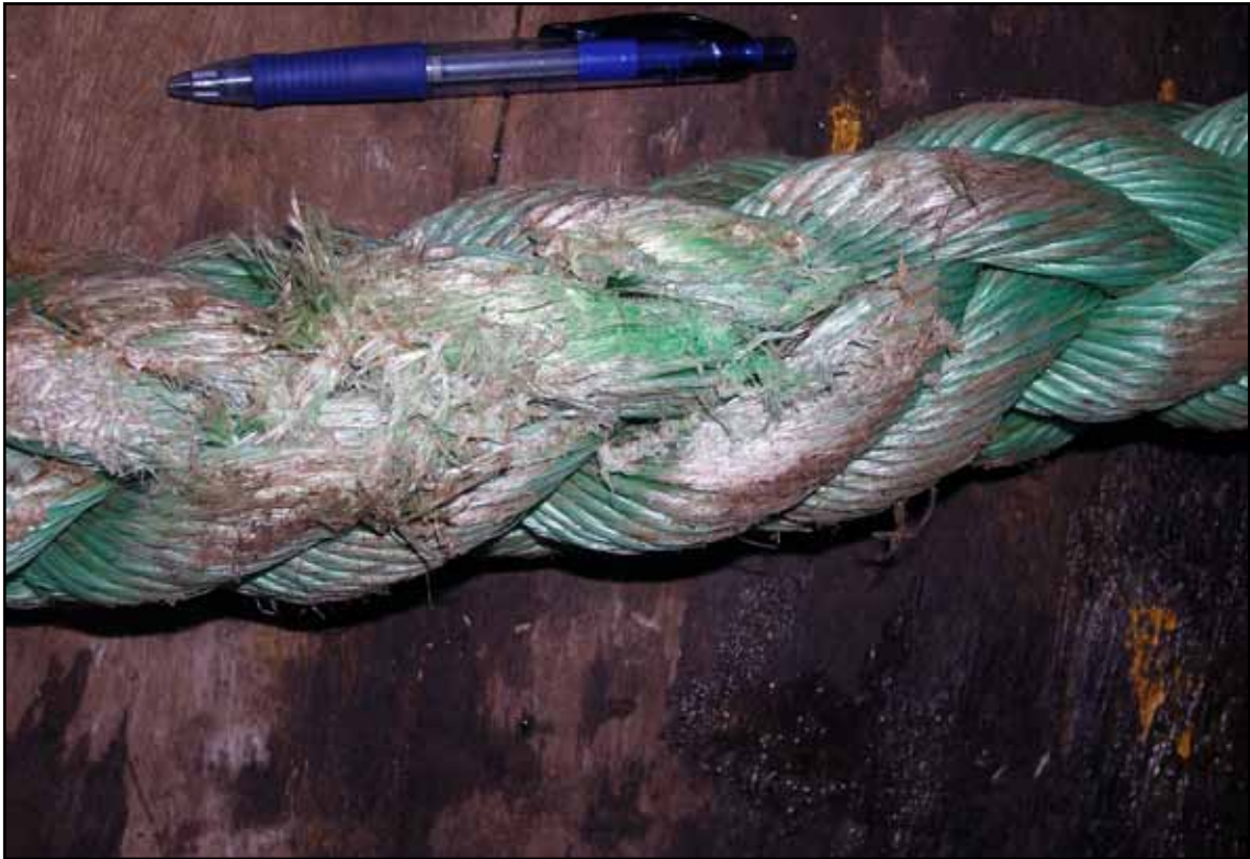
Chafing damage to rope stretcher
