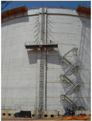
Figure 6 – Access platform at pilaster
