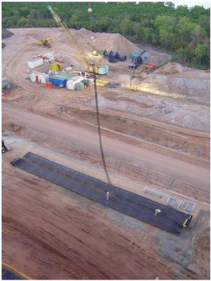
Figure 5 – Installation of prefabricated vertical tendons
