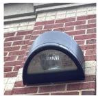
Wall-mounted fixture with metal halide lamp
