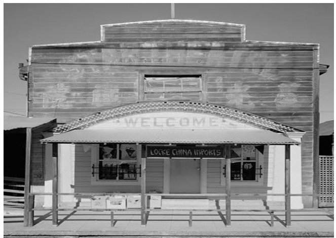
Front façade of Star Theater on River Road. Library of Congress Survey HABS CA-2071-D
