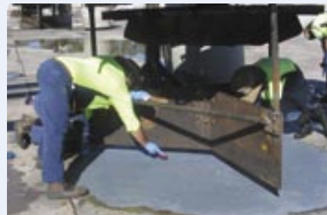
Applying Fixmaster® High Performance Quartz
