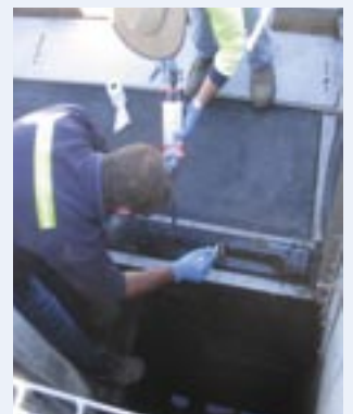
Applying Fixmaster® Rapid Rubber Repair
