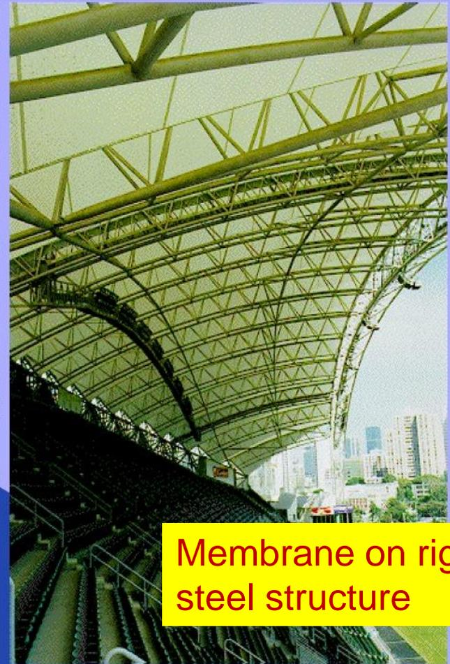
Membrane on rigid steel structure
