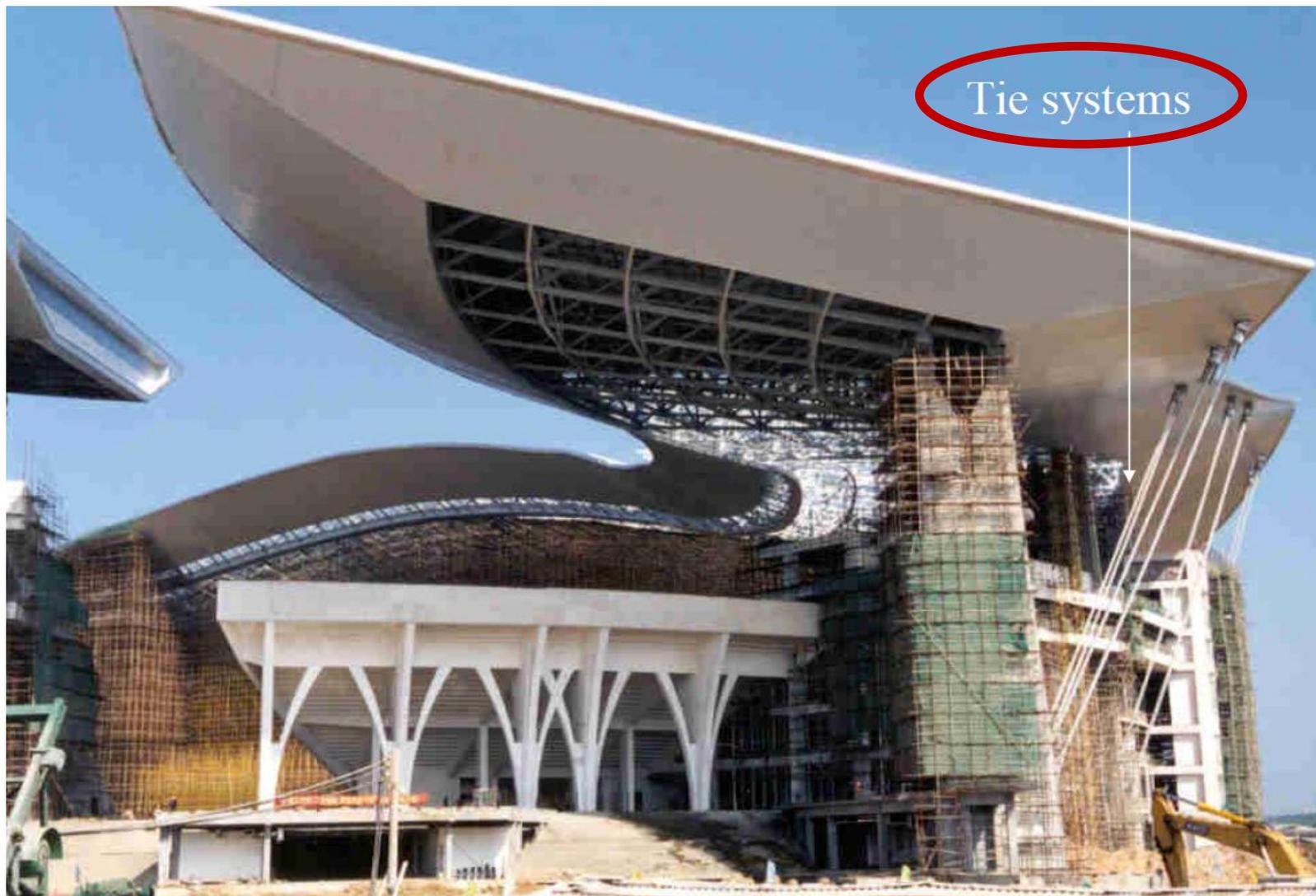
Tie systems to stabilize the cantilevered roof
