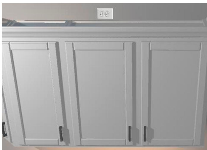
OUTLET ABOVE CABINET
