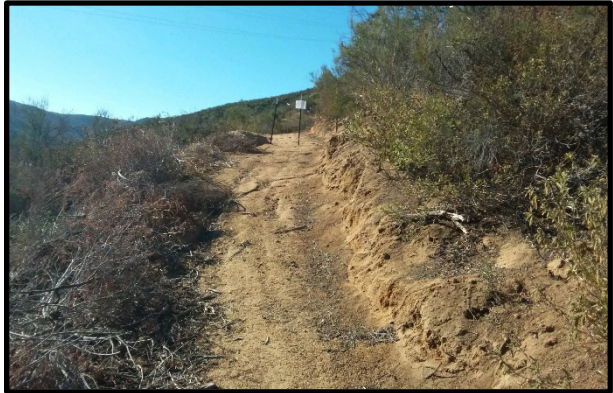
Navajo Bypass reroute closed to stabilize during the winter.
