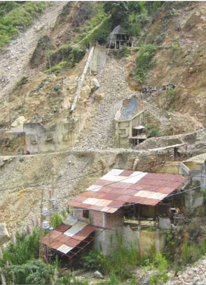
Primitive mining techniques have produced dangerous landslide conditions for local miners. Colombia Goldfields' plan includes moving these people to a safer location...opening the door to mining giants looking for a turnkey operation.
