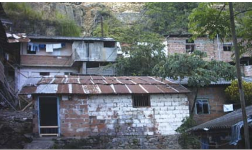
BEFORE work could ever begin, Colombia Goldfields had to ensure the care of families who have been mining Marmato for generations. These are the tin-roof shanties they used to live in.
