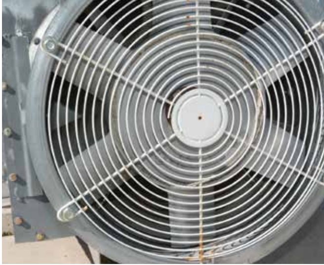
Fig. 8-1. Axial flow fan.
