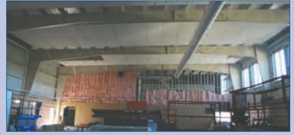
Minter Bridge: interior construction
