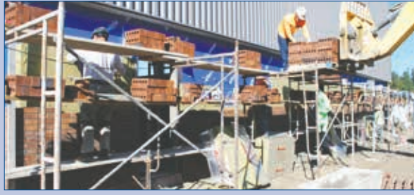
W.L. Henry: bricklaying of exterior wall
