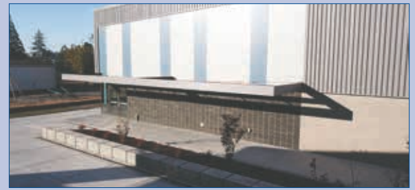
North Plains: the front entry area
