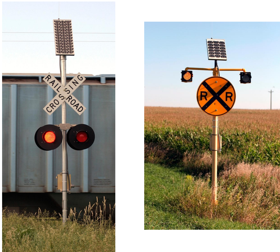
Figure 4-5. Typical Crossing and Advanced Warning Installations
