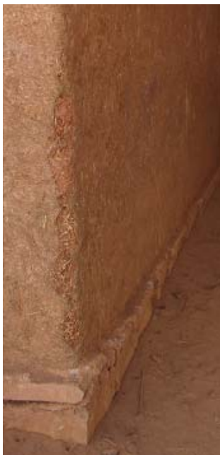
Picture 22. Damage of the mud plaster due to fair wear and tear. [5]
