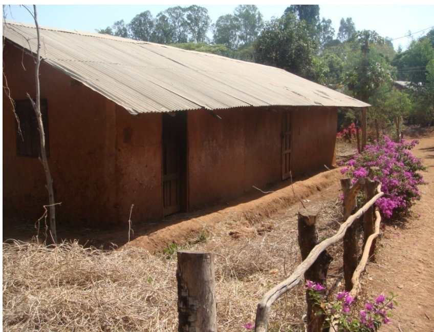
Picture 19. The oldest mud block house in Challia. This roof has protected this house for the last 19 years. The inclination and the ditch protecting the foundation from water are also to be noted as well as the fence surrounding the house keeping livestock out of the yard. [5]
