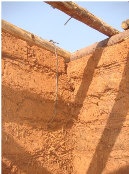
Picture 18. The roof is being secured to the house with reinforcement wires. [5]
