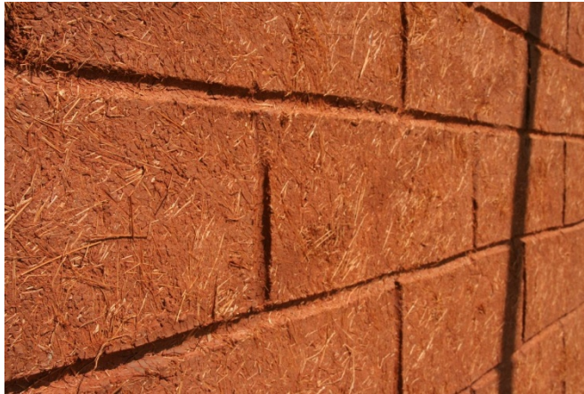
Picture 20. Accurately plastered mud block wall. [18]
