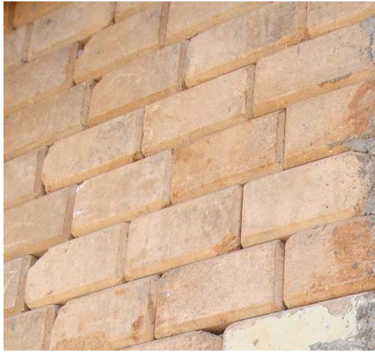
Picture 15. The appearance of a CSSB wall. This wall is constructed of interlocking CSSB hence no mortar is needed. [5]
