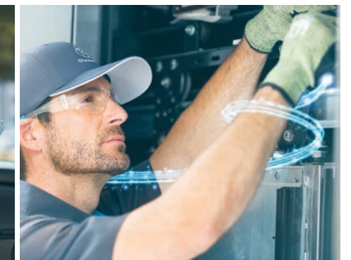
Repairs are completed in less time.
