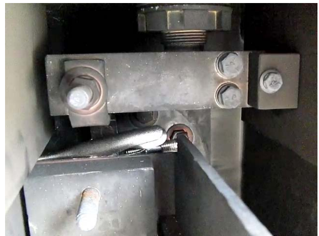
Fig. 5 Vice grip wedged AΦ – BΦ in back of the protector
