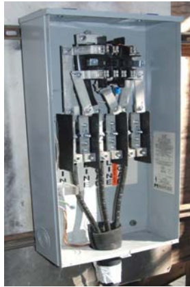
Fig. 15 200-A meter socket with bottom entry and exit
