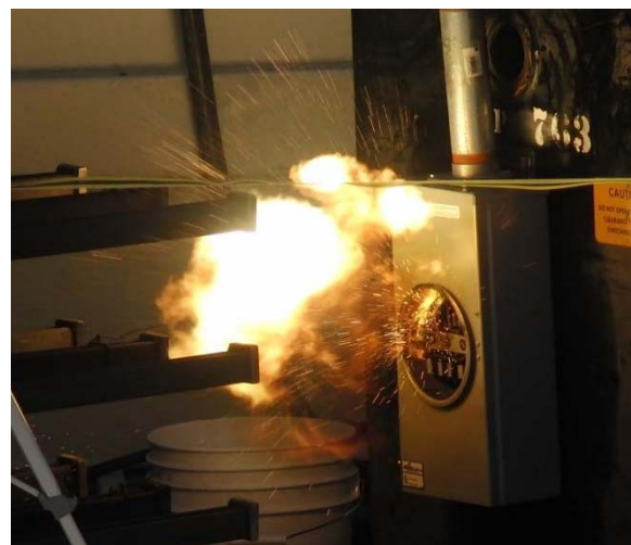
Fig. 3 Example fault on 120/208-V meter socket
