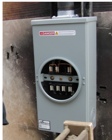
Fig. 8 Ringed self-contained meter socket
