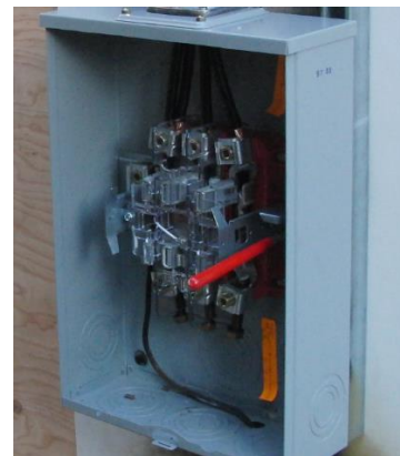
Fig. 14 Ring-less meter socket with cover removed
