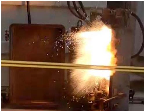
Fig. 4 Example fault on a 208-V network protector
