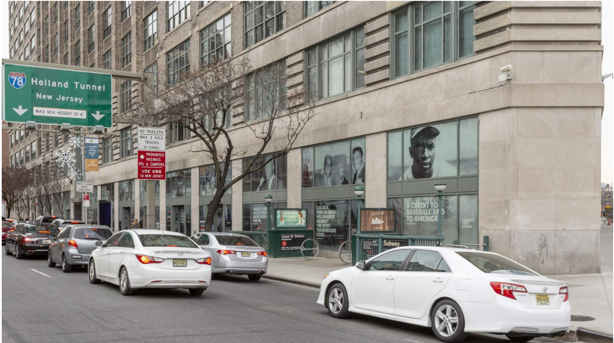
75 Varick Street | Holland Plaza Building (now One Hudson Square) Jackie Robinson Museum LPC Submission V.2 January 15, 2019
