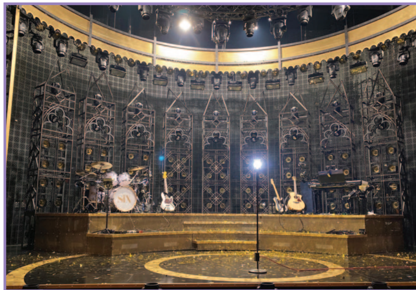
The pixel frames are placed downstage of the curved mesh screen consisting of LED pixel tape.
