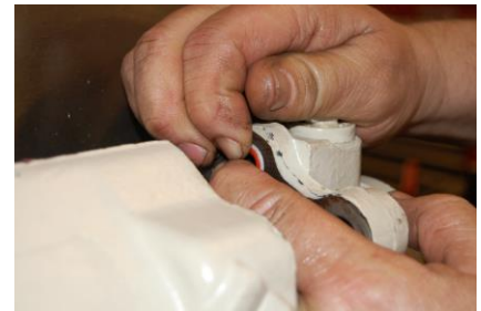
INSTALL NEW TETRA SEAL
