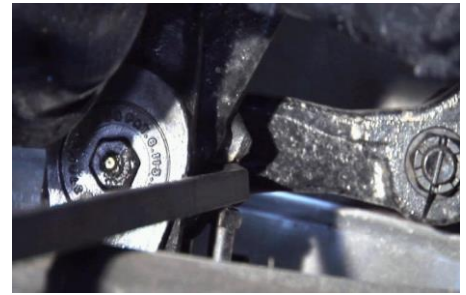
1" BAR USED TO CHECK INTERNAL LEAKAGE
