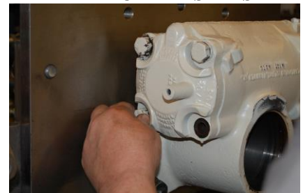
INSTALL AND TORQUE BOLTS
