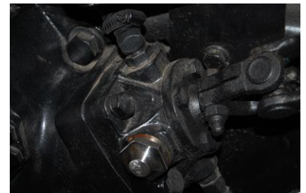
TEST PLUG INSTALLED
