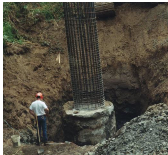
Excavate upper portion of shaft and repair defect area.
