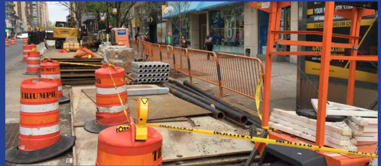
Photo 5: E 86th Street and 3rd Avenue
