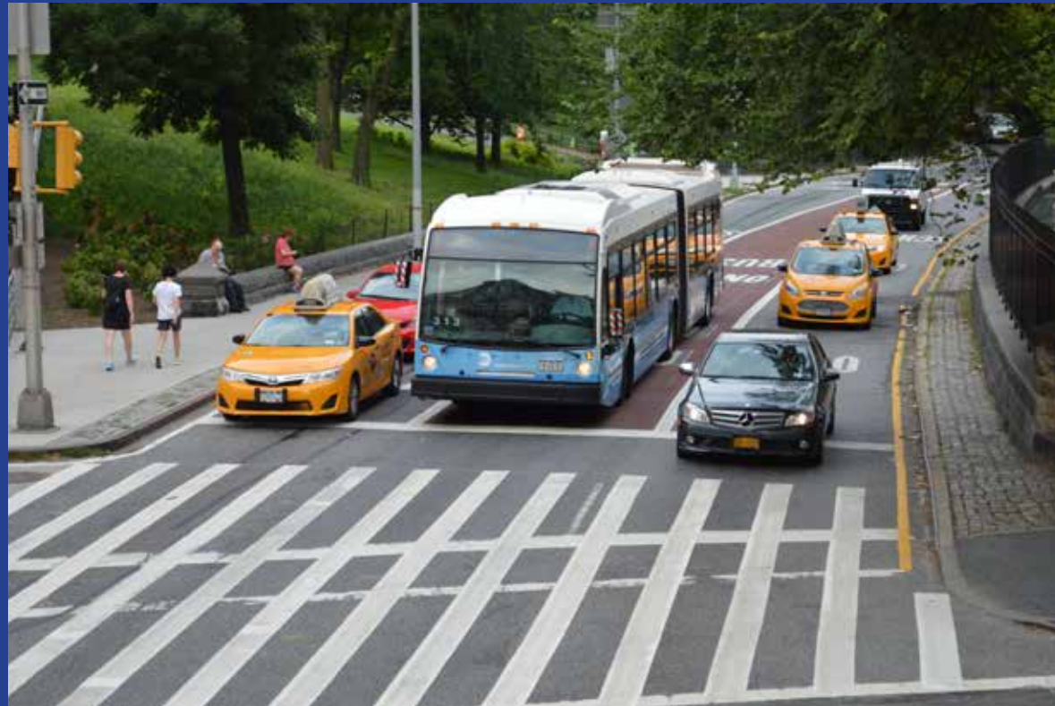
Photo 2: Queue Jump Lane on Eastbound Transverse Road at 5th Avenue
