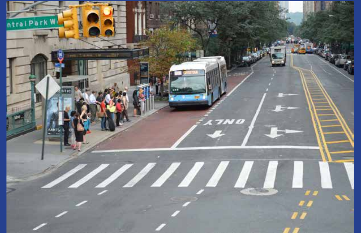
Photo 1: Queue Jump Lane on Eastbound E 86th Street at Central Park West
