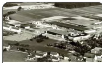
Production plant in Kirchdorf
