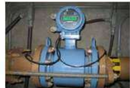
Figure 1. Rosemount 8732E Magnetic flowmeter with SMART Meter Verification.
