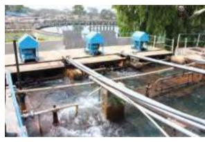
**Oxygenation :** Air and water are allowed to mix with the help of pumps. This causes oxygen from the air to dissolve in the water.
