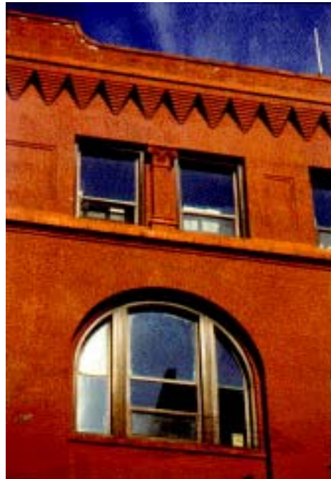
The Main Building and Machinery Hall both possess fine detailing and craftsmanship in sandstone, brick and terra cotta. Top: A detail of fourth-floor windows on the Main Building, ornamented with Romanesque-style attached columns, foliate capitals and impost blocks, and a continuous drip molding. Above left: The Main Building's entrance with a Romanesque-style arch carved with the name "Armour Institute." Left: One of the decorative impost blocks ornamenting the Main Building's entrance arch. Above right: Machinery Hall is detailed with Classical-style pilasters and brick corbeling.
