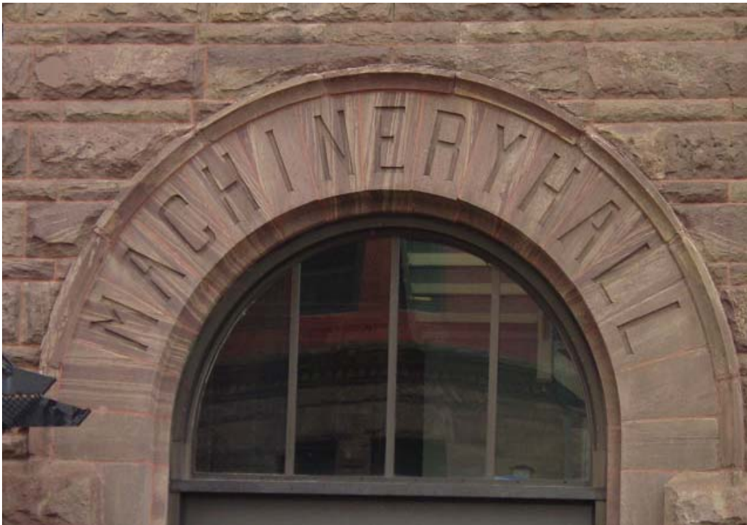
Both the Main Building and Machinery Hall are fine examples of the Romanesque Revival style, possessing the important characteristics of the style, including round-arched entrances and windows and medieval foliate ornament. Top: An upper-floor detail of the Main Building. Above: The main entrance to Machinery Hall.
