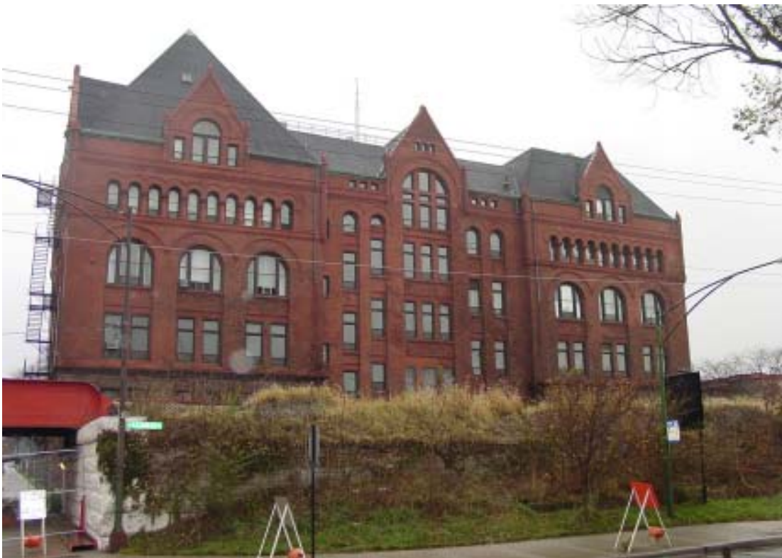
The Main Building from the northeast (top) and northwest (above).
