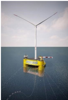
Figure 6-6. Floating WindDesal module for 30,000 m 3 /d [31]
