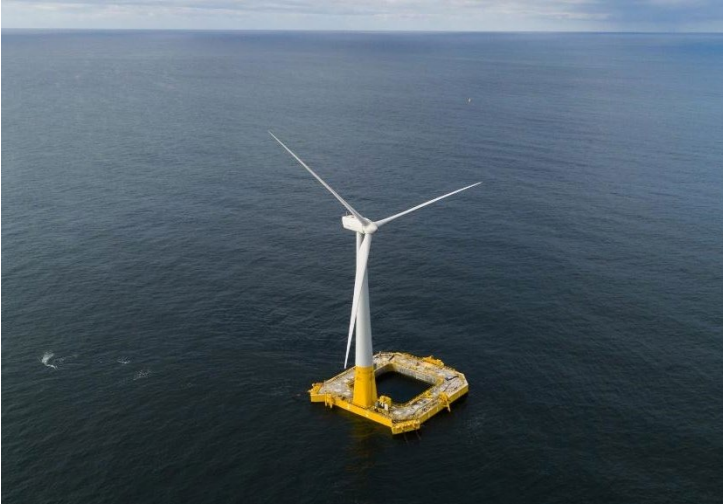
Figure 5-2. BW Ideol's barge hull concept design
