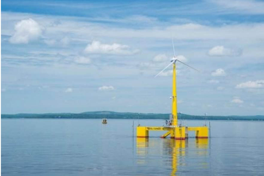
Figure 5-1. University of Maine floating semi-sub 1:8 scaled prototype
