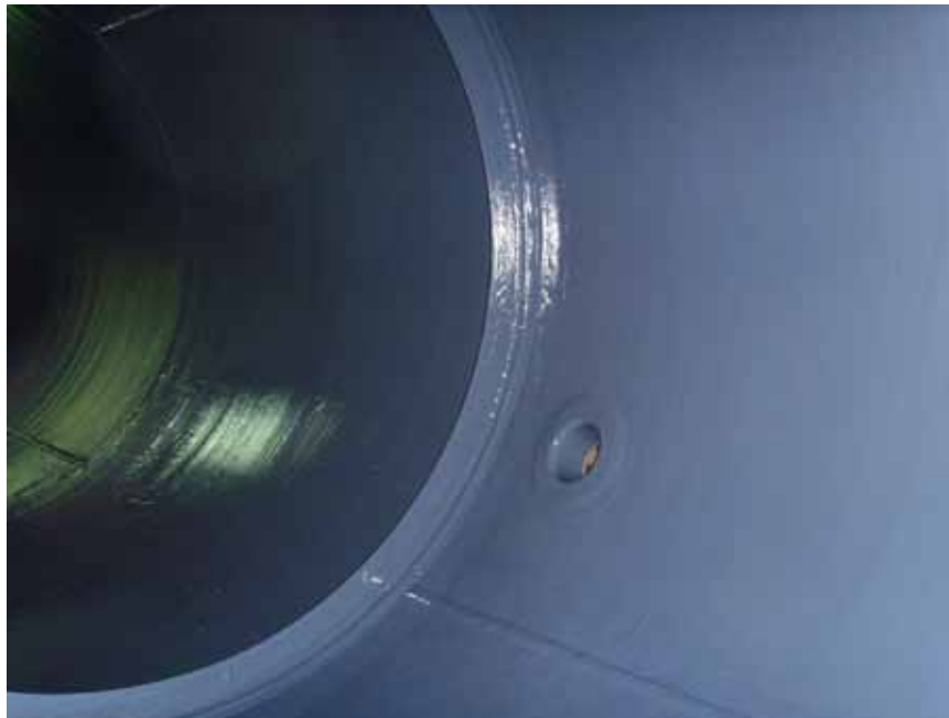
Belzona lining applied to a newly fabricated separator
