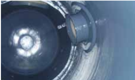
100% solids epoxy protective linings for erosion-corrosion protection
