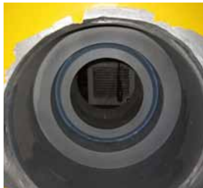
Bush installation, North Sea
