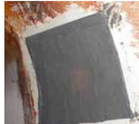
Glass flake lining repair
