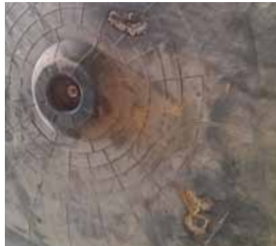
Deteriorated fender
