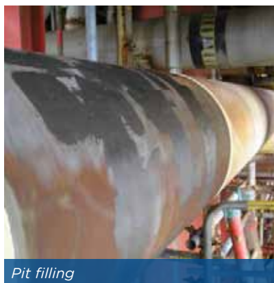
Corrosion under insulation
