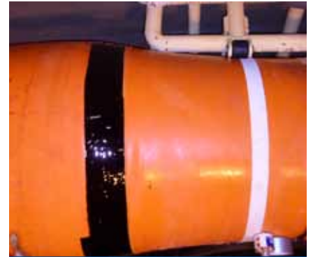
Belzona flexible repair
