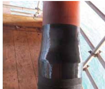
Corrosion repaired and cladding sealed
