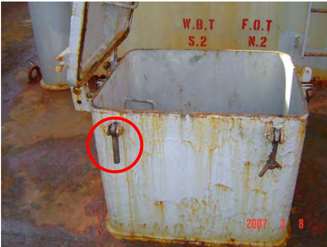
Missing nut of small hatch
