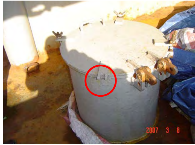
Missing nut and bracket
