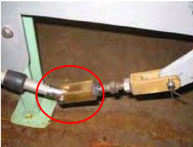
Incorrect condition of turn buckle
