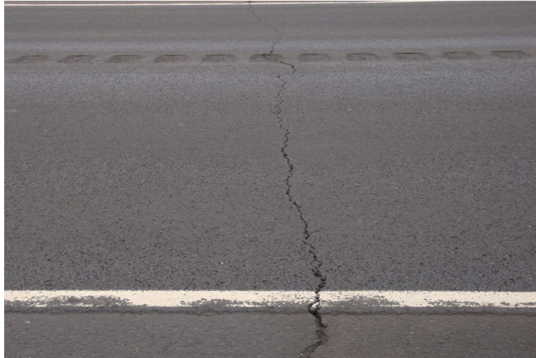
Exhibit 3-2 Transverse Cracking
