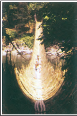
Figure 6.7 : Rope Bridge (Arunachal Pradesh)
