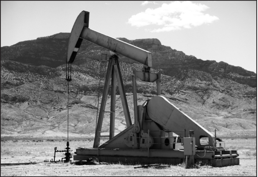
Pumpjack for the Sand Dune 88-35 oil well in the Sand Dune Oil Field, Nye County (Lowell Price photo).
