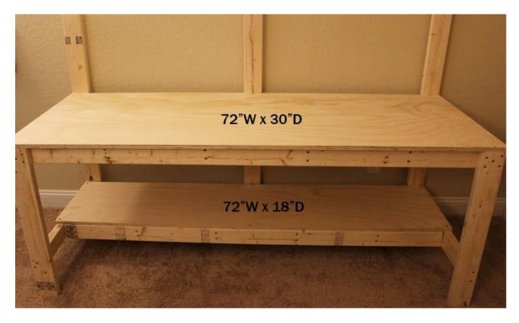
After the horizontal pieces of plywood are secured, go ahead and attach the back panels to the frame.
