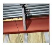
FROTH-PAK™ Foam Insulation is ideal for sealing areas 6" wide or less (max. 2" thick) and can be left exposed per NFPA 286 in roof/wall junctures.
