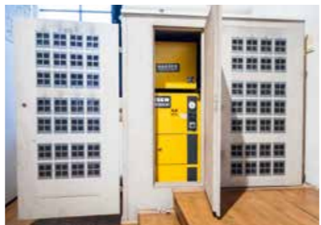
A KAESER AIRBOX is responsible for controlling the stops in the great organ
