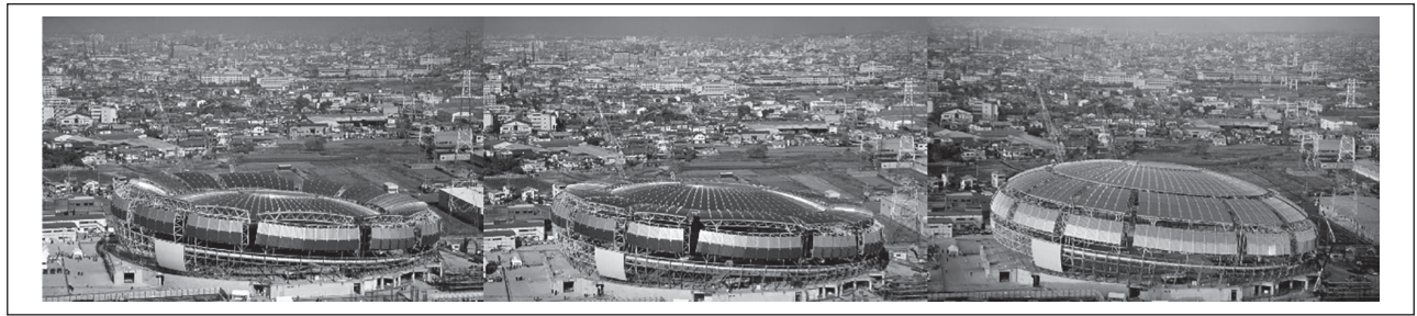
Image 9. Deployment of the Namihaya Dome, Kobe (1996). Courtesy of Kawaguchi & Engineers.
