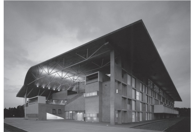
Image 6. Aira Gymnasium, Kagoshima (2004). Photo credit: Hiroshi Hito, Nikkei Architecture, 31 October 2005. Courtesy of Kawaguchi & Engineers.
