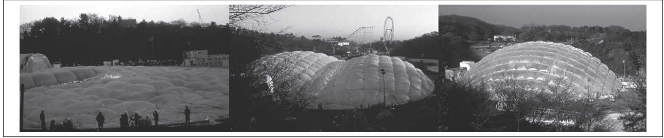
Image 8. Inflation of the 12th World Orchid Conference Pavilion, Kanagawa (1987). Courtesy of Kawaguchi & Engineers.
