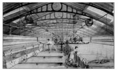
**In 1783** Richard Arkwright's steampowered mill on Miller Street was Manchester's first cotton factory, taking cotton spinning out of the home and turning it into a mechanised industry.
