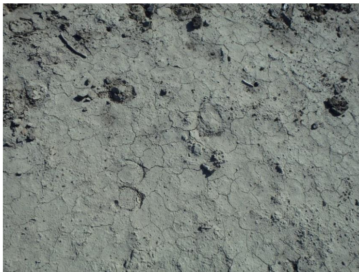
Figure 13. Shrink-swell cracks covered with fine-grained silt or clay, characteristic of hydric clay soils.
