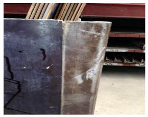
With the box loosely assembled, tighten Z nuts with hammer, ensuring all the while that the rebate on the shutter aligns with the steel corner.
