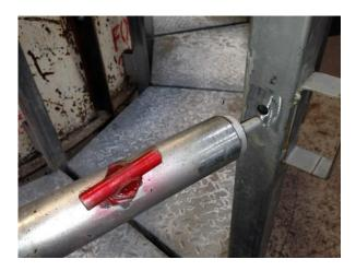
Loosen locking nut so that length of telescopic rail can be adjusted. Insert pins of rail into pre-drilled holes.
