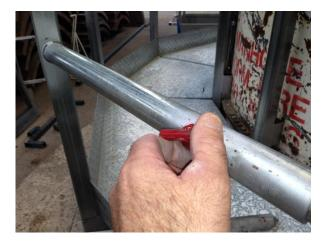
Extend telescopic rail to maximum length and tighten nut. Repeat for every rail, one top rail and one middle rail.
