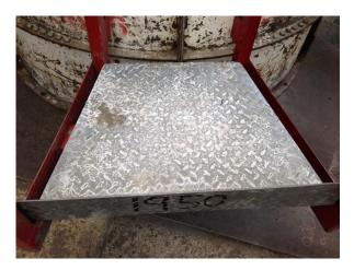
Locate the plate in between the 2 red brackets, narrow end first, lowering the kick board end and adjusting the location of the red brackets as required so that the folded edges of the floor plate sit loosely against the joists. **The structure is safe to take your weight now.**
