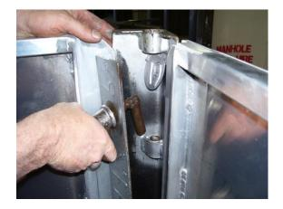
Loosen Z nuts so that clamping plate is removed far enough from corner to allow the placement of panels.
