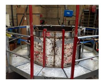
The assembly is complete. It can be lifted into place by securing appropriate rigging to **lifting lugs** located on each outer form panel.
