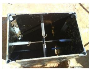
Using the braces supplied put in position and wind out until they are firm against the inside of the pit.
