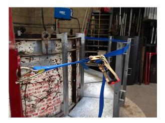
Secure one end of the tensioning strap to a lug at either side of the entry. Thread the strap through each and every eyelet and secure to the lug the other side of the entry. Tension until the upright brackets have no loose play. **The tension strap is not a physical restraint**, its sole purpose is to prevent movement whilst balustrade parts are fitted.
