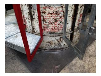
The rest of the hanging brackets and floor plates may be added, one at a time, ensuring all the while the brackets are hanging vertically and each plate has minimal play. If the last plate to be fitted is too loose, or tight, the hanging brackets can be adjusted one way or another by a slap with your hand or take a firm grip on any bracket and give it a shake sideways.
