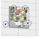
Manually screw the cylindrical guides into the holes in the box.
