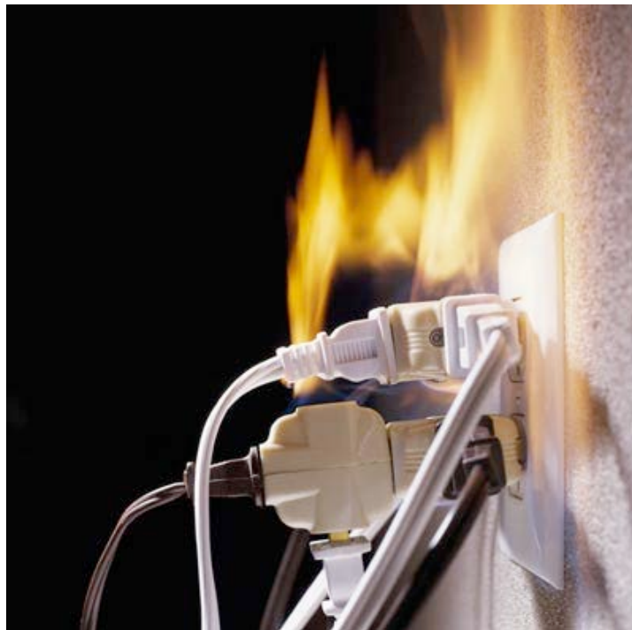
Figure 2 Example of an overloaded electrical outlet
