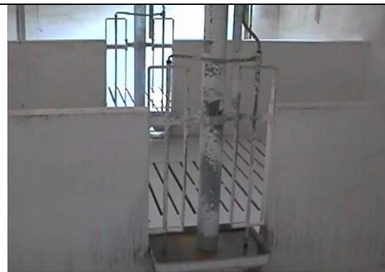
Lime-wash used as the terminal disinfectant in a grower house
