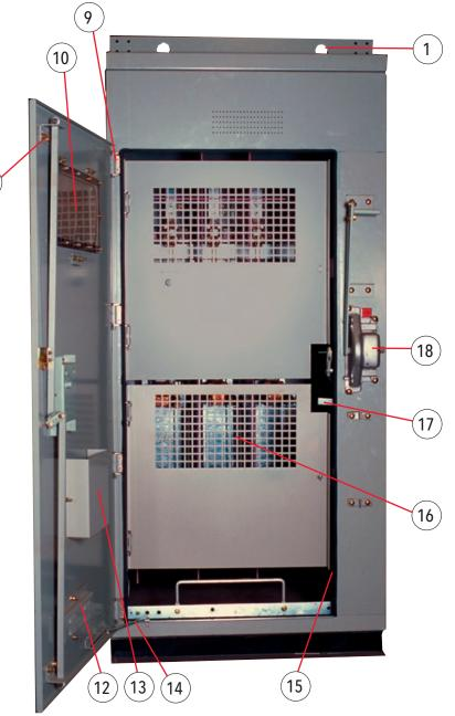
Enclosure door is open to show internal screens with openings for viewing switch position and blown-fuse indicators.
